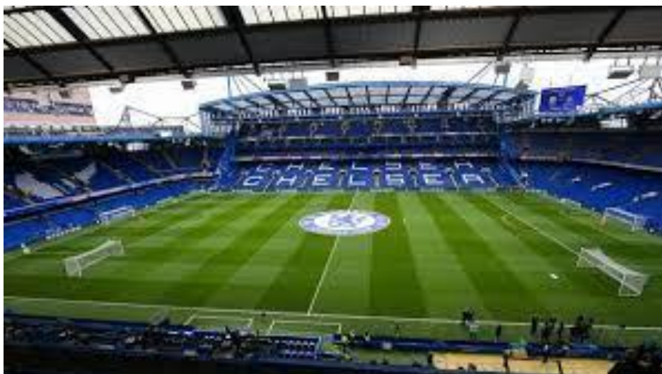
New Stamford Bridge Stadium - Chelsea
