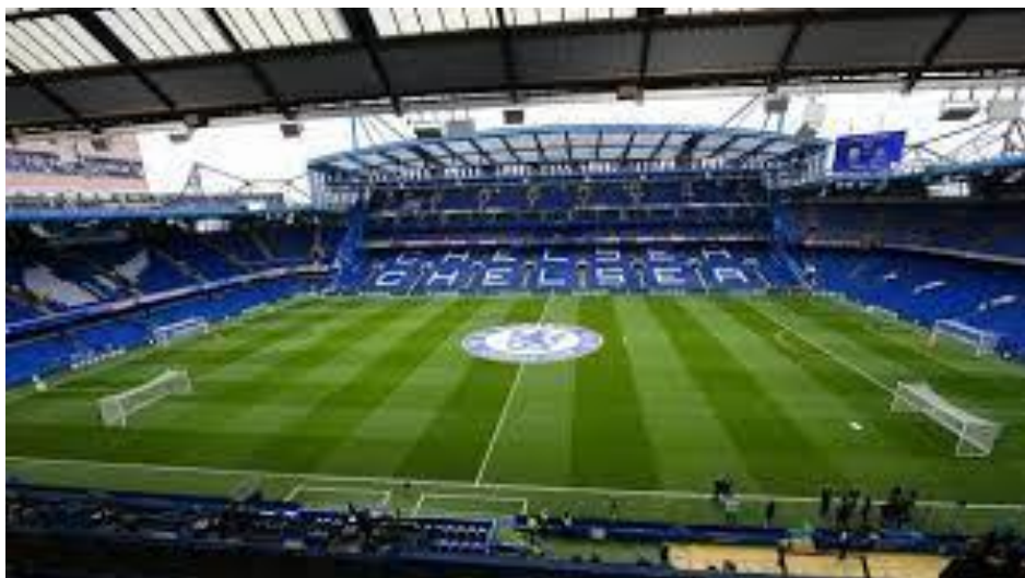
New Stamford Bridge Stadium - Chelsea
